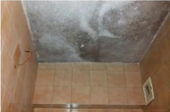
**Before application:** ceiling in sanitary facility infected with fungi and mould. Visible dark spots.
